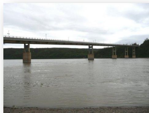
Yukon River Bridge
