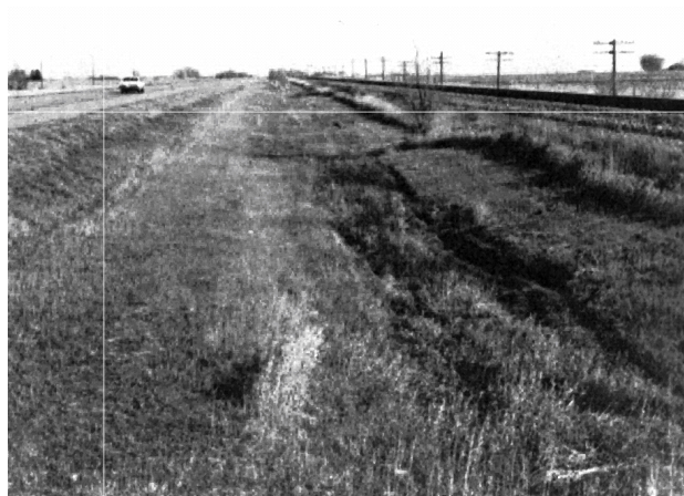
Figure 1160-2 Rural Roadside Hazard Rating of 2
