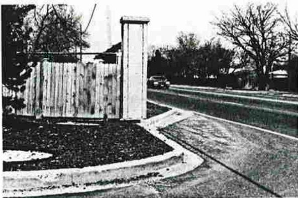
Poor corner sight distance can adversely affect gap acceptance and stopped approach capacity.
