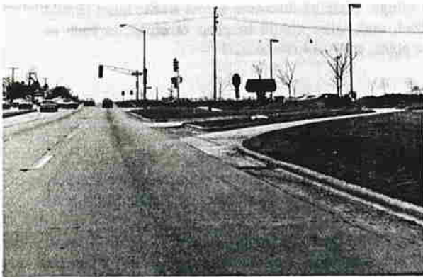
Note the offset of the center island from through traffic lanes.
