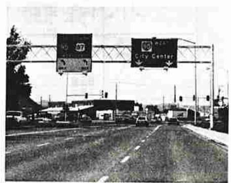
(c) Advance signing is important at high-volume intersections with double turning lanes.
