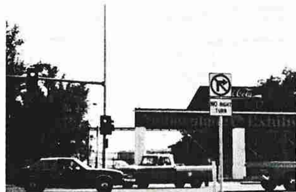
Small (less than 5-foot) corner radii serve to discourage undesirable right turns.
