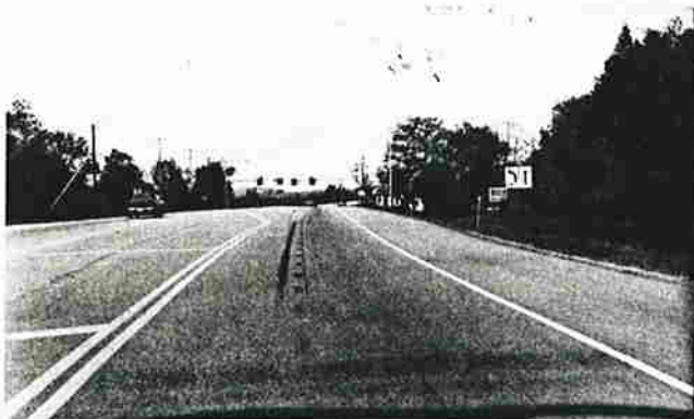
Long approach tapers and lane lengths are necessary to provide for safe deceleration for turning vehicles.
