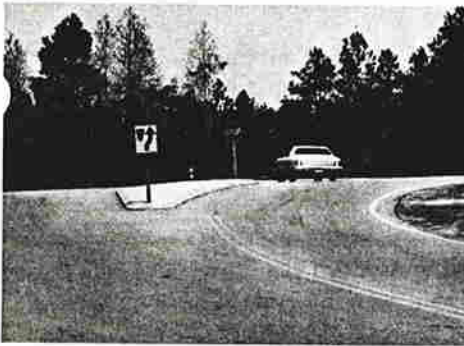
(a) The eastern approach of Route 70 is brought in at right angle and stop-controlled. The median island stores a stop sign and provides separation from opposing turning vehicles. Note the offset of the median nose from the painted centerline.
