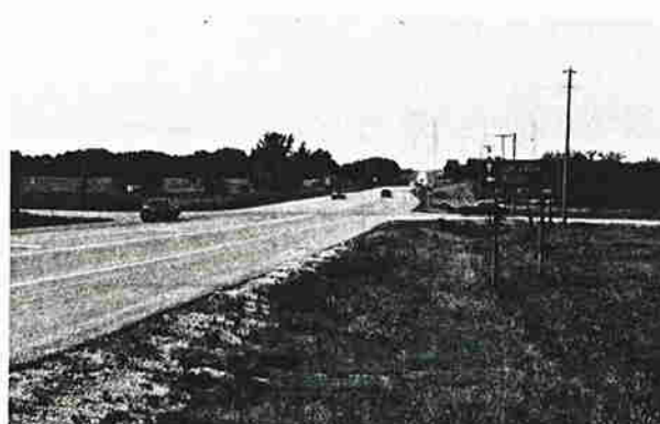
Stop controlled intersections on high-speed highways must be designed with adequate sight distance.
