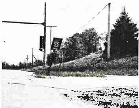
(d) The corner islands are offset a full lane width from the edge of the through lane.
