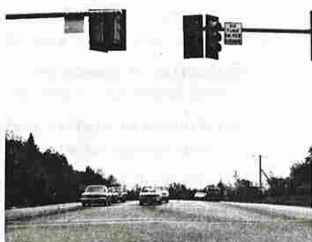
(f) Note the great crossing distance and open pavement area created by the skew angle. The installation of traffic signals provides a means of reducing exposure to crossing conflicts within this intersection.
