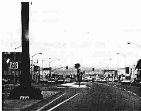
(b) The roadway transitions from a narrow to an 18-foot median. This 18-foot dimension is adequate for full-width left turn lanes, and protection/refuge for pedestrians at the intersection.
