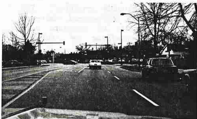
Left turn lanes facilitate signal phasing.
