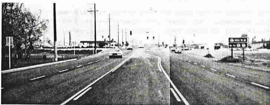
(c) The re-designed intersection scheme emphasizes treatment of left turns rather than right turns.
