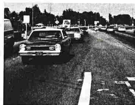
(b) The short left-turn lane from State Route 178 was frequently blocked by queues.
