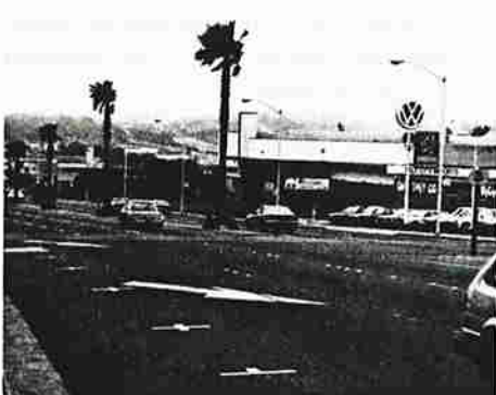
(e) The widened median necessitates merging of three through lanes into two. Large pavement arrows assist in the transition.
