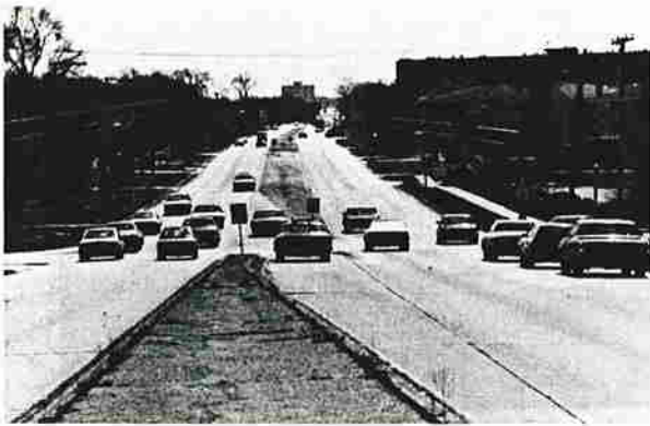
Channelized left turn lanes and exit legs separate points of conflict and define vehicle paths, thereby greatly simplifying the left turn movement.
