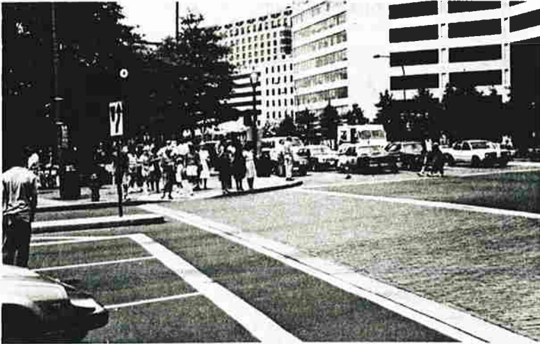
Offset ramp on wide crosswalk.
