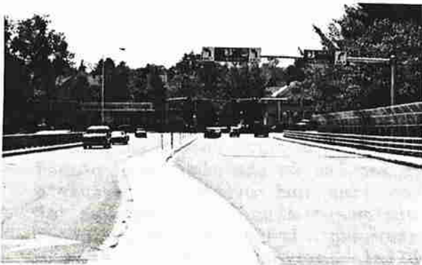
Major turning movements should be delineated with channelization, pavement markings and signing.
