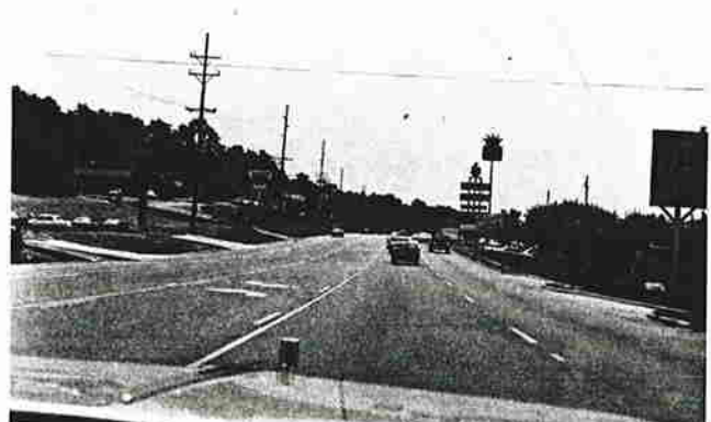
Continuous two-way left turn lanes promote safe access to multiple driveways outside higher speed through lanes.
