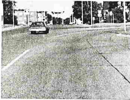
(a) Before construction, eastbound traffic on U.S. Route 10 encountered large open pavement, with no protection for vehicles bound for Frazee Street. The continuity of U.S. Route 10 is not clearly defined.
