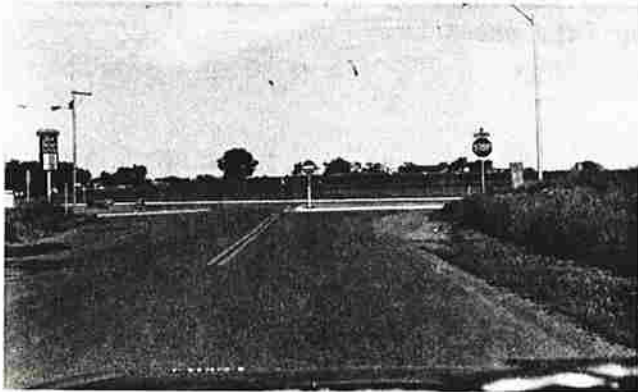
Physical islands or raised medians block undesirable movements.
