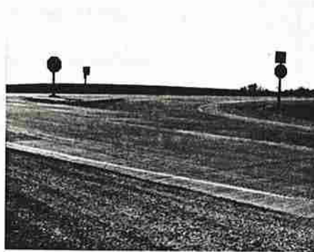
b. The channelization enables large truck turns, separate storage of one queued left turning vehicle, and placement of stop signs within the driver's cone of vision.
