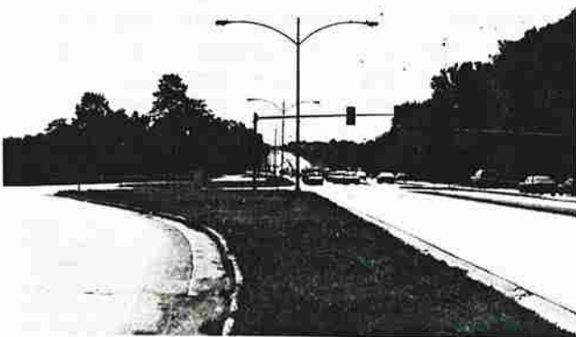
Separation between frontage roads and through arterials eases the driver's task of handling multiple conflicts.
