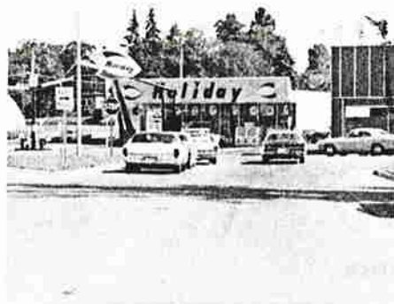
(b) Before construction, westbound U.S. Route 10 was forced to stop at Frazee Street.
