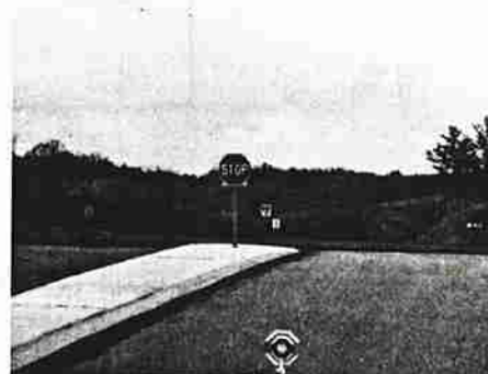
(b) The median island is used to post stop signs.
