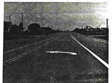
(b) and (c) The design of the left turn lane requires turning vehicles to make a positive maneuver into the lane. Pavement arrows confirm the lane designation.
