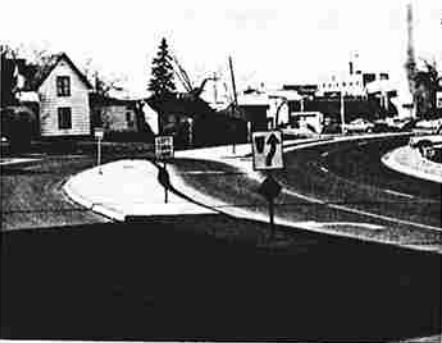
(d) After reconstruction, the through continuity is well defined. Storage for left turning vehicles improves both safety and efficiency of the through movement.
