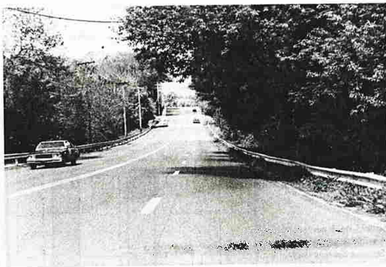
Extension of the channelization taper (above) provides the only visual cue of the intersection over the crest of the hill.
