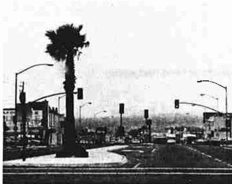
(a) The new median fully protects the left turn lane on the northbound approach to the intersection. Note the use of raised pavement markers, which are common to California.
