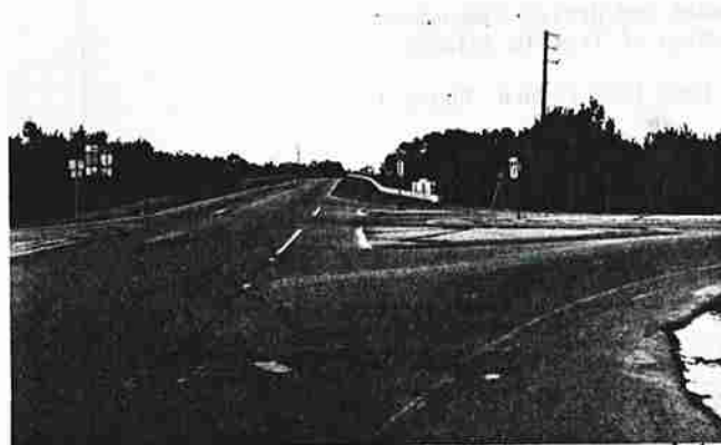
Note the continuous tapering effect created by careful placement of both corner islands.
