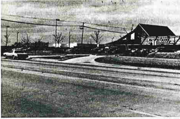
Both curb radius design and width promote easy turns off the arterial.
