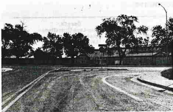
Note the offset of the center island. Islands can be used to prohibit unsafe or undesirable movements.
