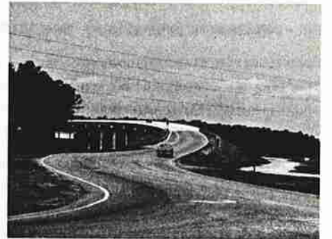
(b) and (c) The new alignment provides good sight angles to both legs for drivers at the stop line. Note the cleared roadsides which provide sufficient corner sight distance.
