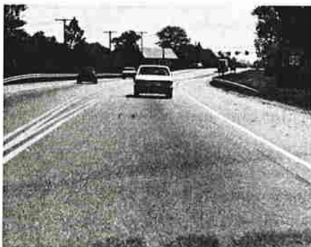
(a) The approach taper for the left turn lane begins in advance of the horizontal curve.
