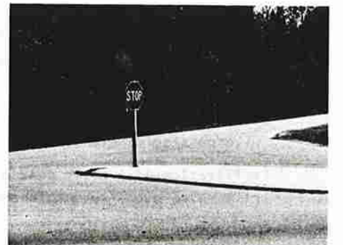
(f) The mountable, raised median island also serves as a visual cue of the intersection, yet does not represent an impact hazard to errant vehicles.
