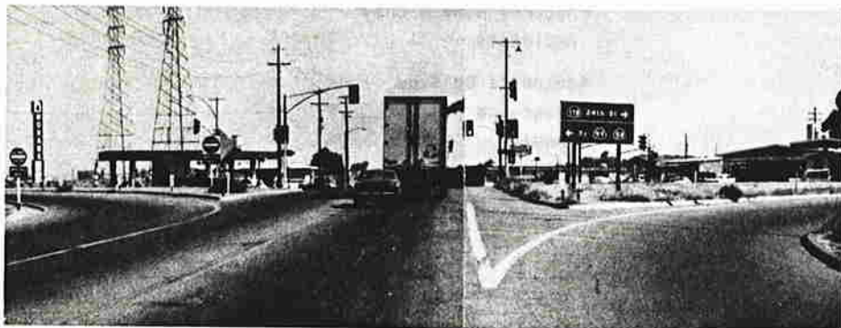
(a) Prior to redesign, the intersection channelization scheme emphasized free right turn movements to and from Oak Street.
