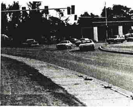
(a) Auxiliary pavement markings and a wide throat assist the movement of the double left turn from the east leg.
