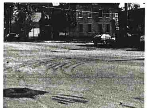
(f) The proposed design will eliminate this wide open intersection, and better define all traffic movements.
