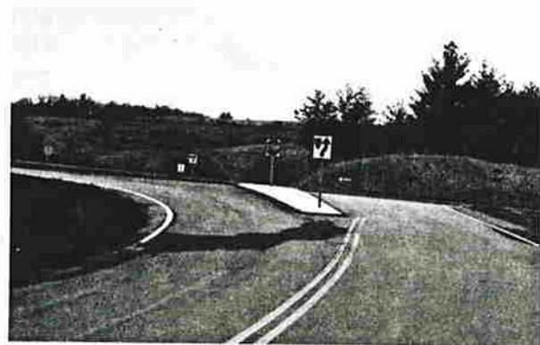
Channelization should clearly separate opposing traffic flows.
