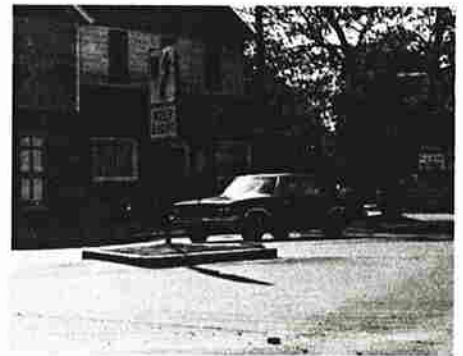
(c) The triangular traffic island in the middle of the intersection serves no channelization function.
