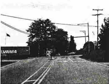
(e) Lane arrangements on the minor approaches reflect traffic volume patterns. Opposing volumes and left turn volumes are low enough to combine left and through traffic in a single lane.
