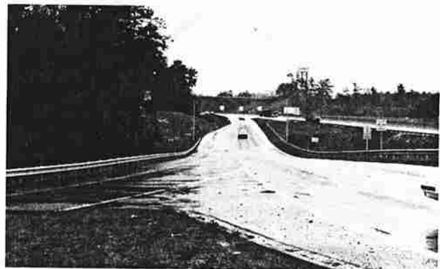
Turning movements and through lanes are clearly delineated with the use of tapers, pavement markings, and arrangement of lanes.
