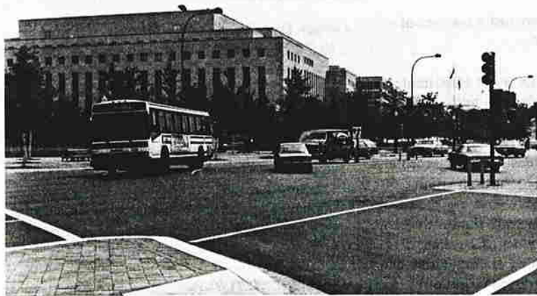
Wide throat widths enable comfortable placement of vehicles turning two abreast.
