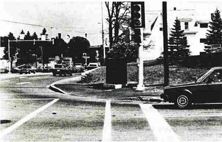
Centered ramp on small radius curb return. Note the placement of the traffic signal and controller, which provide a clear area for pedestrians and wheelchairs.
