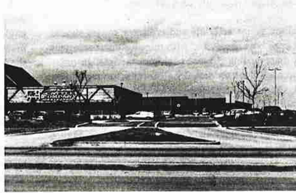
The double driveway is particularly applicable to high traffic generators such as restaurants.
