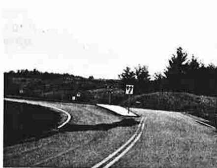
(a) Raised median channelization on the minor approach separates opposing movements and provides a visual cue of the intersection.
