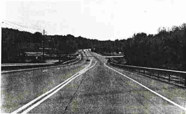
Turning movements and through lanes are clearly delineated with the use of tapers, pavement markings, and arrangement of lanes.
