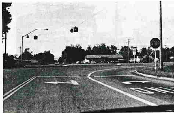
Right turn movements are generally easier than through and left turns, as traffic from the right does not interfere with the turn.
