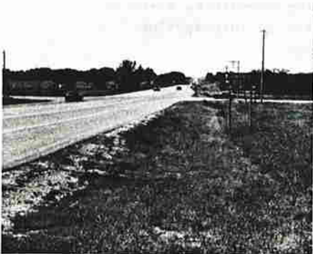
(d) Excellent sight distance is available in all quadrants of the intersection. All signs were relocated inside a 1500-foot sight line on the approaches to U.S. Route 24.
