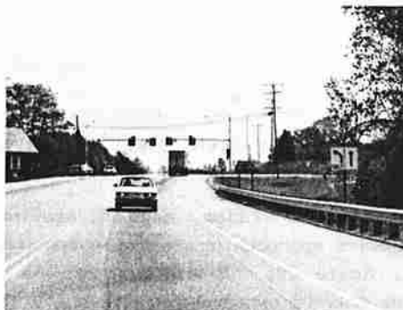
(b) View of approach from the west. Note the fully shadowed left turn lane and visibility of overhead traffic signals.
