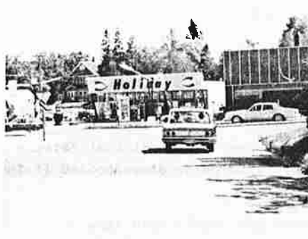
(e) After reconstruction, continuity for westbound traffic is established. Note the stopped vehicle on the Frazee Street approach.
