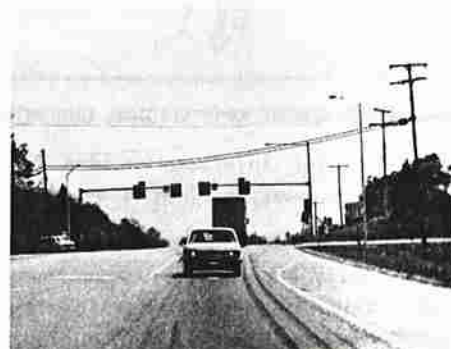
(c) Right turn lanes are developed for the acute angle turn despite the low demand volumes. The angle requires a very low speed turn, hence the need to separate right turns from high speed through traffic.
