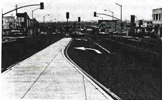
Left turn lanes should be clearly delineated from through lanes.
