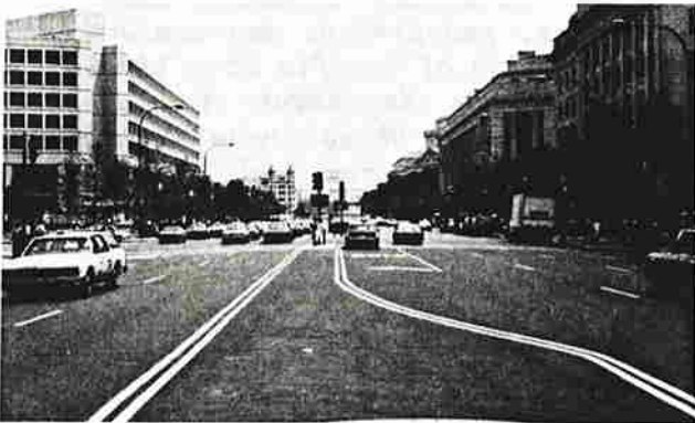
Left turn vehicles awaiting gaps can safely queue within left turn storage lanes.
