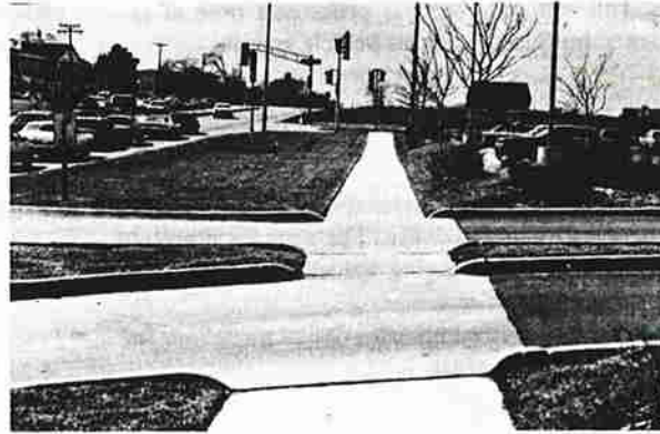
The driveway also accommodates pedestrian movements along the sidewalk.
