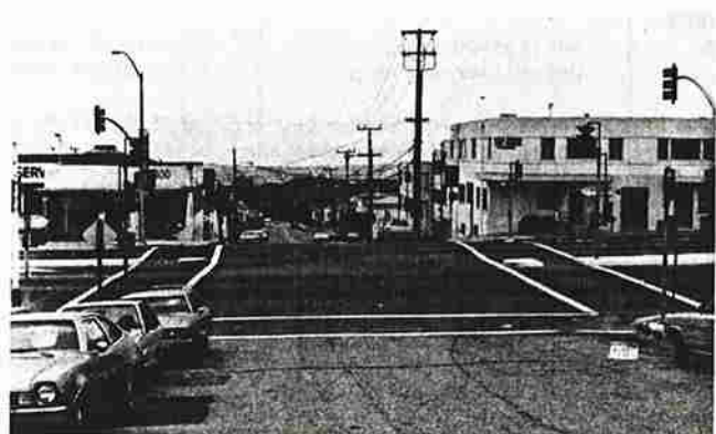
Median design and crosswalk placement can be coordinated to provide refuge to pedestrians and the handicapped. Note the break in the median islands at the crosswalk. This design specifically accommodates wheelchairs.
