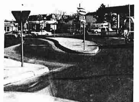
(c) Design of the channelization provides protection for stopped vehicles, clearly defines the through route, and produces conflict angles of about 90°.
