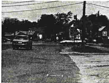
(b) Cross traffic from West Street and businesses along Broadway add conflicts to the intersection and complicate the driving task.
