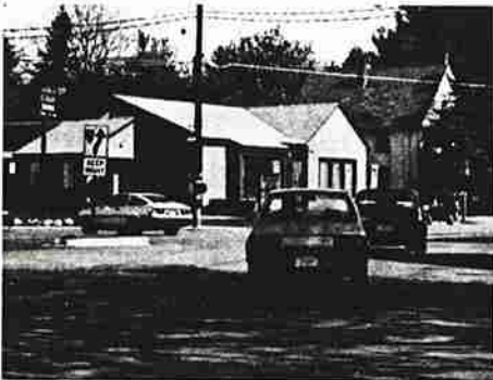
(d) Heavy turning volumes from Broadway to South Street, Broadway to Clinton Street and Clinton Street to South Street create many opportunities for angle, sideswipe and rear-end accidents.
