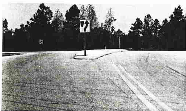
Raised islands are useful for placement of traffic control devices in locations within the driver's normal sight lines.
