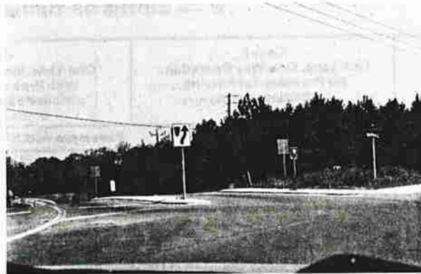
Traffic islands physically separate opposing traffic flows.
