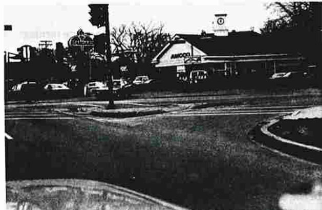
This island is large enough to effectively function as a channelizing island for right turns, a location for pedestrians (note the handicapped ramps) and a location for the traffic signal.
