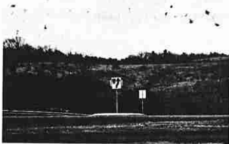
(c) and (d) Raised median channelization is effective in guiding vehicles across the intersection.
