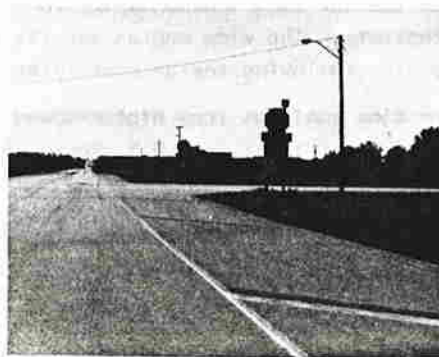
(e) The approaches on U.S. 24 were reduced to one lane, with the former right lane striped out. This 1) provides visual notice of the intersection; and 2) gives a distinctly different appearance to the stopped approach (as in the above photos).
