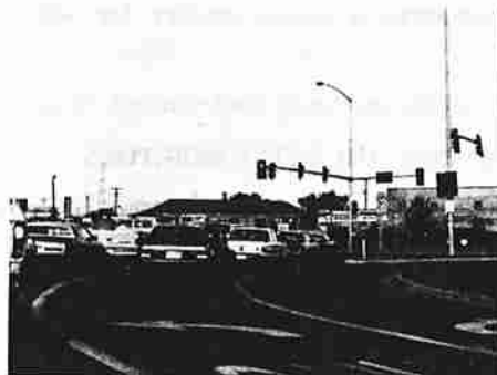
(e) Turning lanes are long enough to assure independent queuing and operation.
