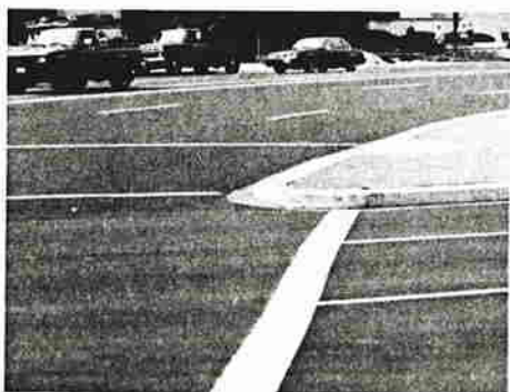
(d) The new angle of intersection of Constitution Avenue is about 45°, which is an improvement over the previously very shallow angle.
