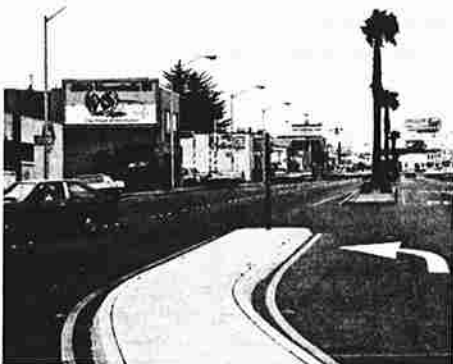
(d) Exclusive u-turn channelization just north of Como Avenue serves southbound traffic from Gambetta and Como.
