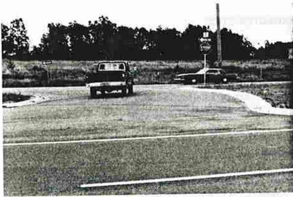
Merging conflicts are created by right- or left-turning vehicles that interact with traffic on the departure leg.
