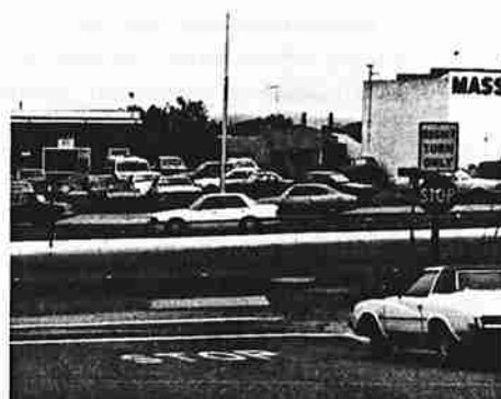
(f) Left turn access at Gambetta Street is eliminated through extension of the raised median.
