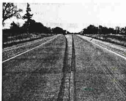
d) and e) The long taper develops a left turn lane for west to north movements.
