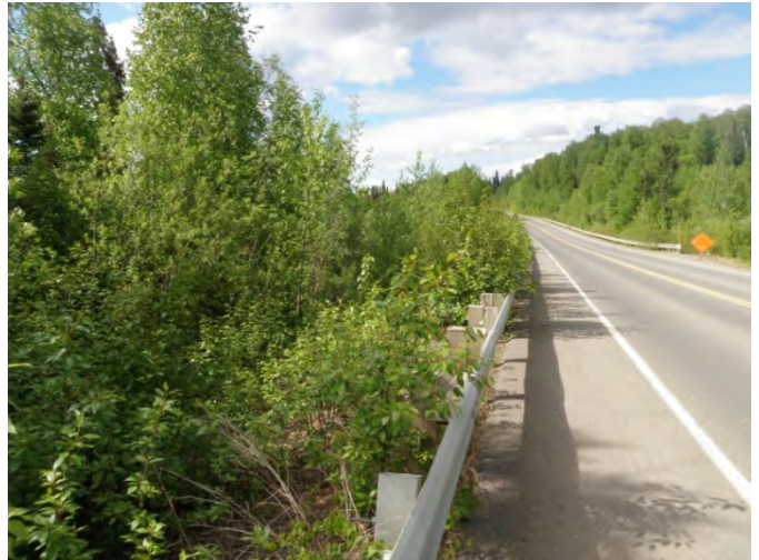
Photograph 3: Vegetation present in Zone 1 and sight lines impaired by woody vegetation in Zone 2.
