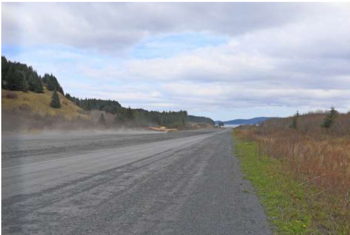
Gravel habitat along runway (N57.88456 x W152.84886)
