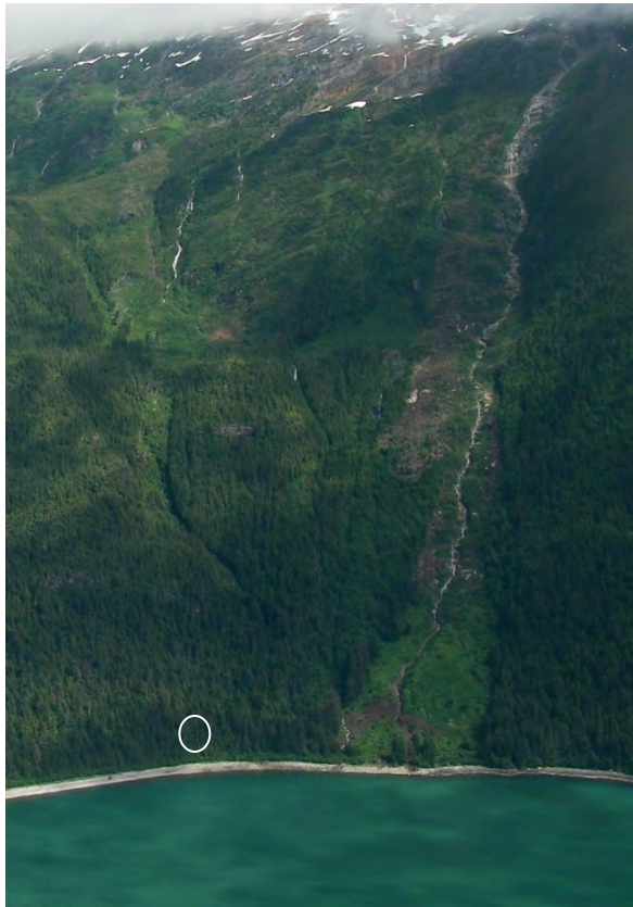
RF10. View east/upslope at rockfall.
