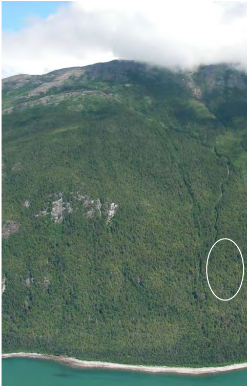
RF12. View east/upslope at rockfall area.
