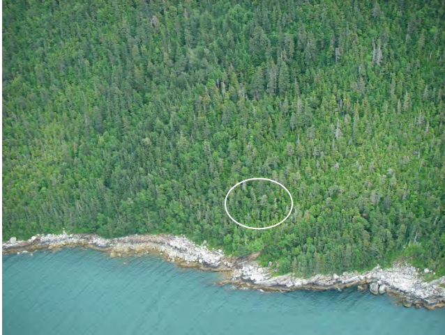
RF16. View east/upslope at rockfall hazard.
