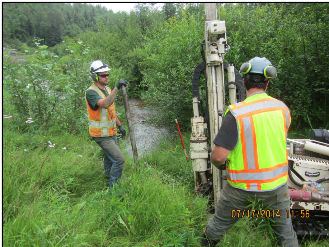
Photograph 22 – Geoprobe set up to drill 19-BH14/19-MW3 near creek on the south side of the highway. View to the south.
