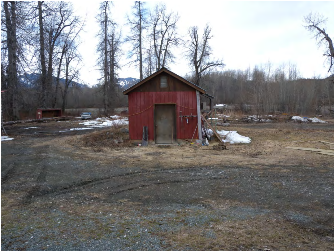
Storage Shed 1 looking W. Unoccupied building with concrete floor (Photographer: Sweet)
