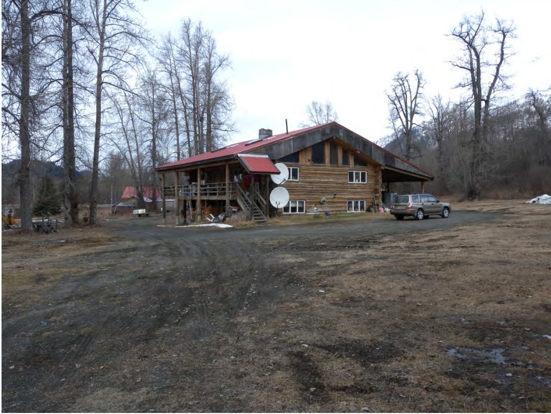
Jacquot House 1 looking S. Occupied building with concrete foundation (Photographer: Sweet)
