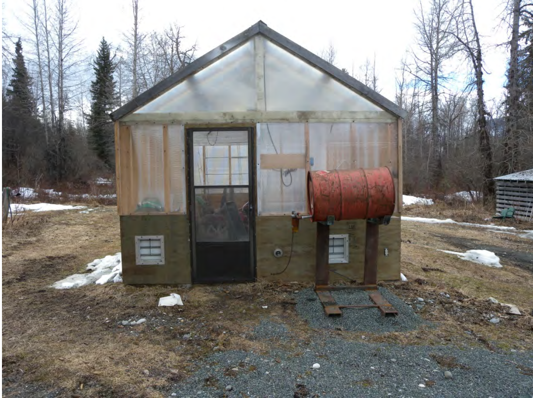
Greenhouse building looking S. Unoccupied building with gravel floor (Photographer: Sweet)
