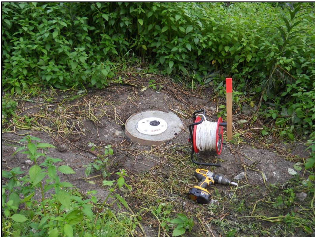
Photograph 28 – Flushmounted well completion - 19-MW2. View to the south.
