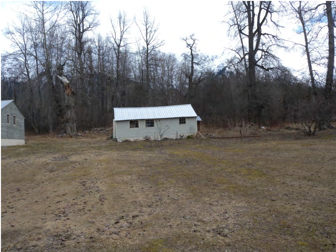
Storage Shed 2. Unoccupied building with wood floors. (Photographer: Sweet)
