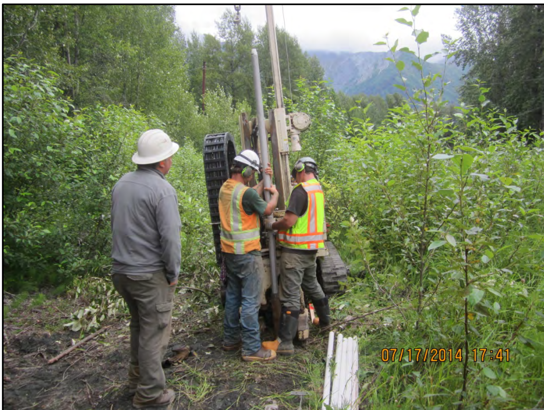
Photograph 48 – Geoprobe installing well 25-MW1 in boring 25-BH08. View to the west-northwest.
