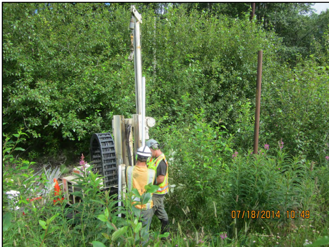
Photograph 40 – Setting 25-MW2, steel pole marking valve box visible to on right-hand side of photograph. View to the northeast.
