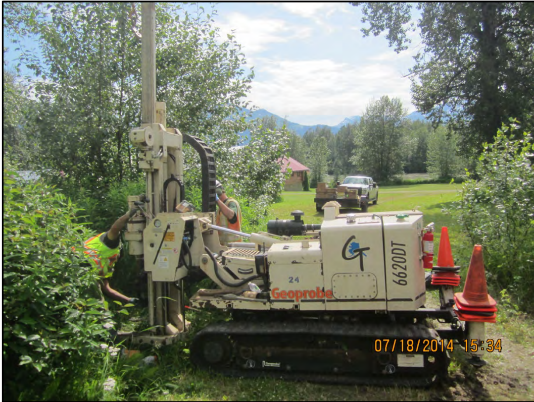
Photograph 41 – Geoprobe drilling boring at 25-BH14/25-MW3 location; view of house in the background. View to the southwest.
