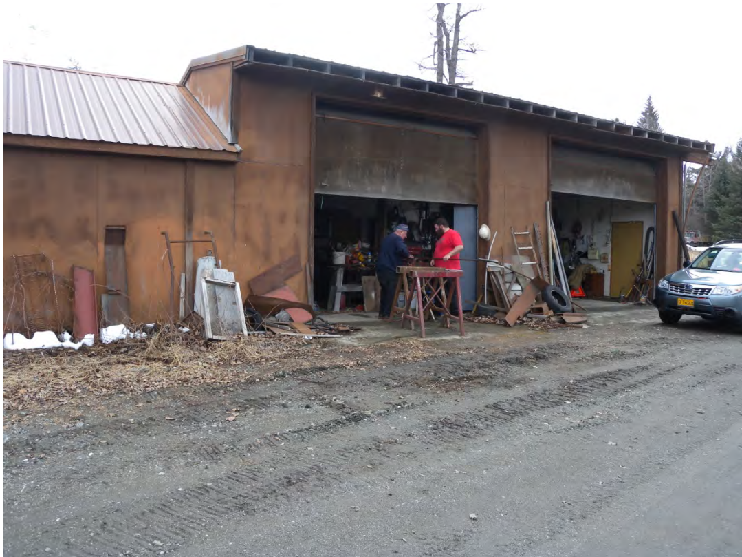
Shop/Storage Building looking E. Unoccupied building with concrete foundation (Photographer: Sweet)
