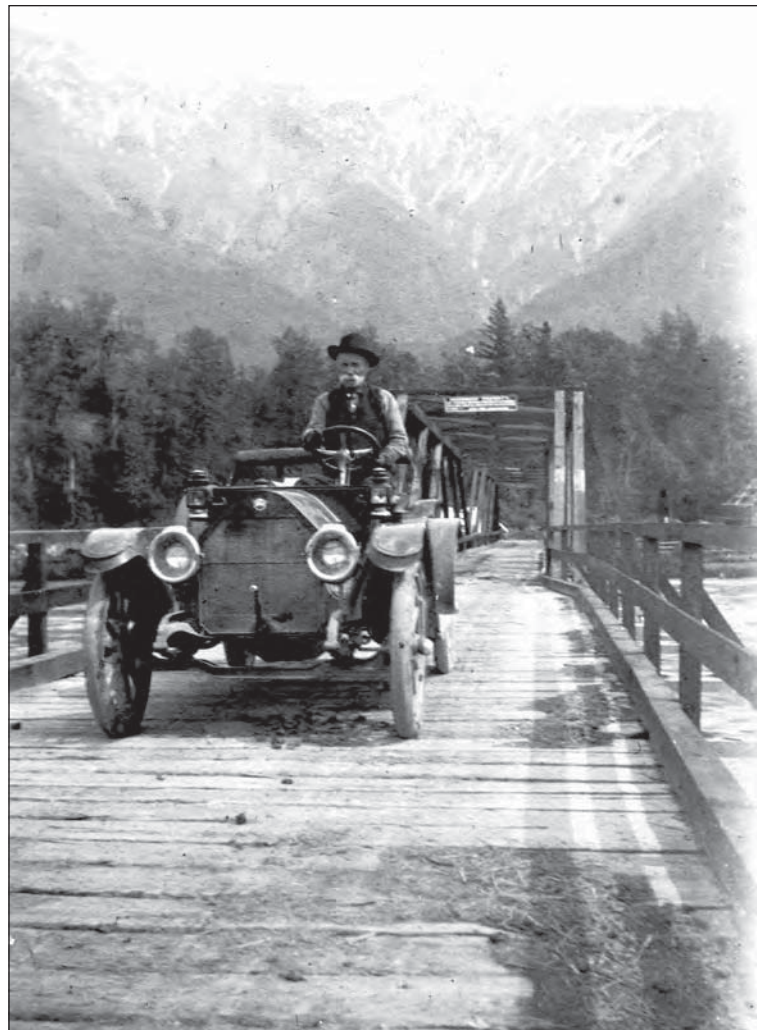
Figure H-6. Vehicle on the first Wells Bridge showing the through truss Howe spans.
