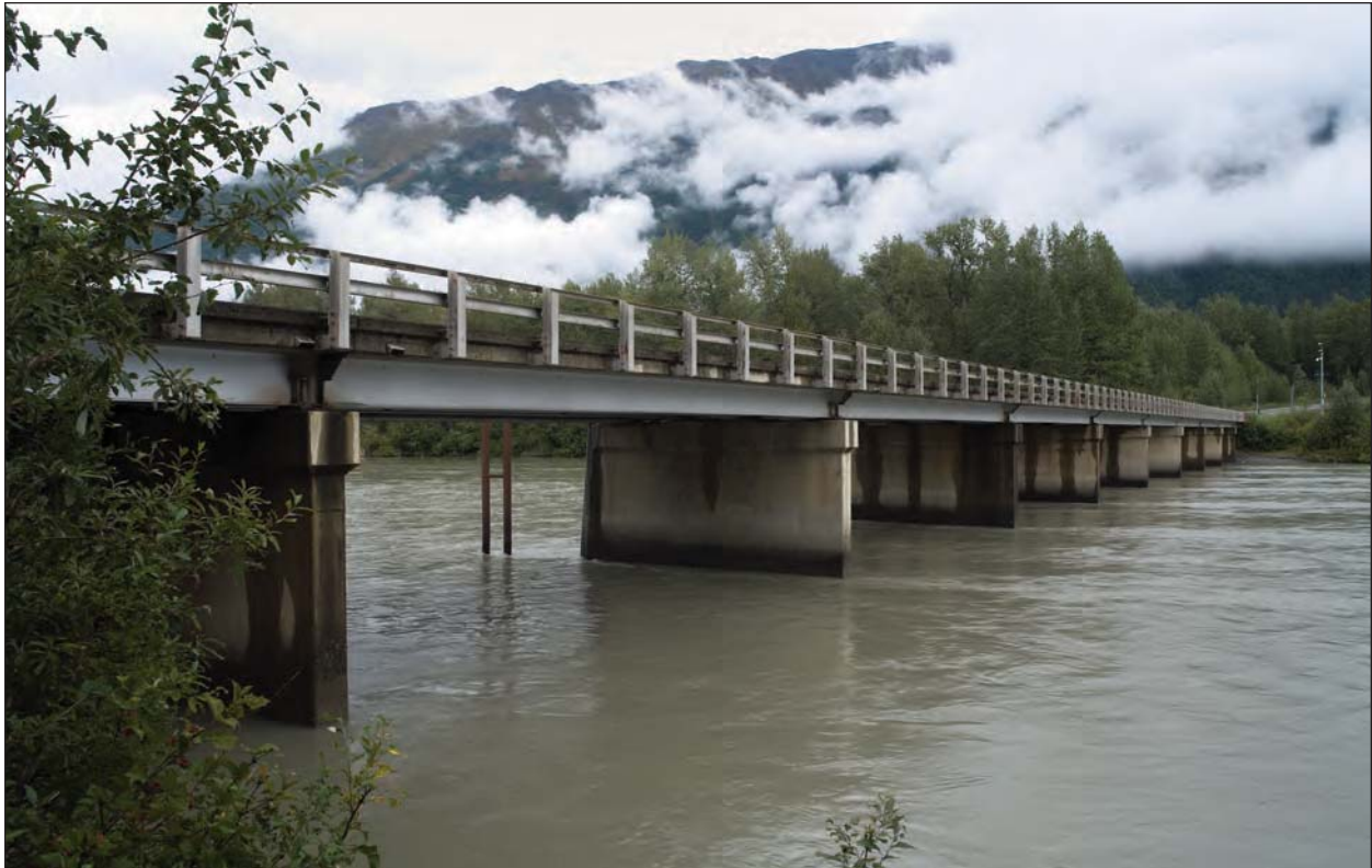
Figure H-12. Downstream side of bridge looking southward toward Haines. .
