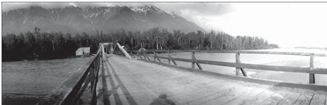
Figure H-3. King-post span installed on the first Wells trestle (SKG-548).
