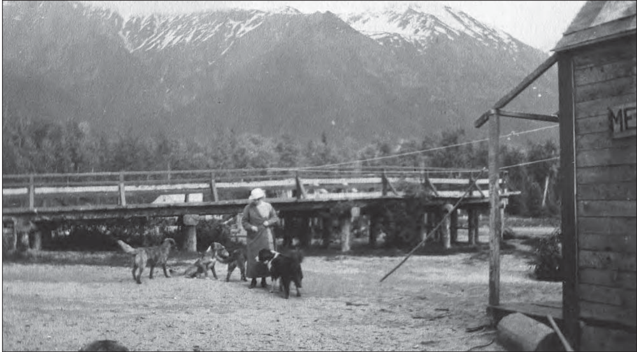
Figure H-4. Northern end of the first Wells trestle showing the curve at the northern bank of the river.
