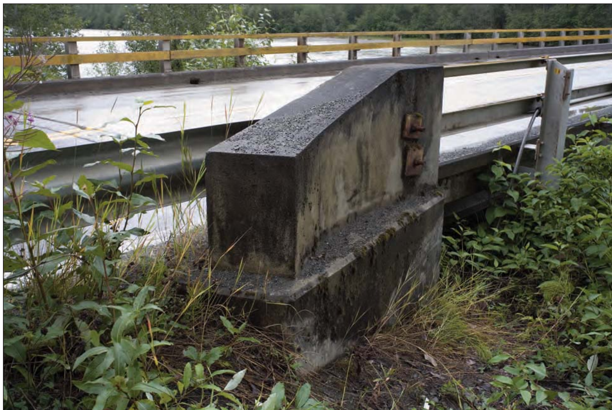
Figure H-18. Formed concrete approaches and safety railings.
