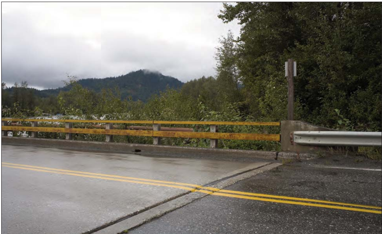
Figure H-15. Yellow-painted safety railing and concrete deck and curb.
