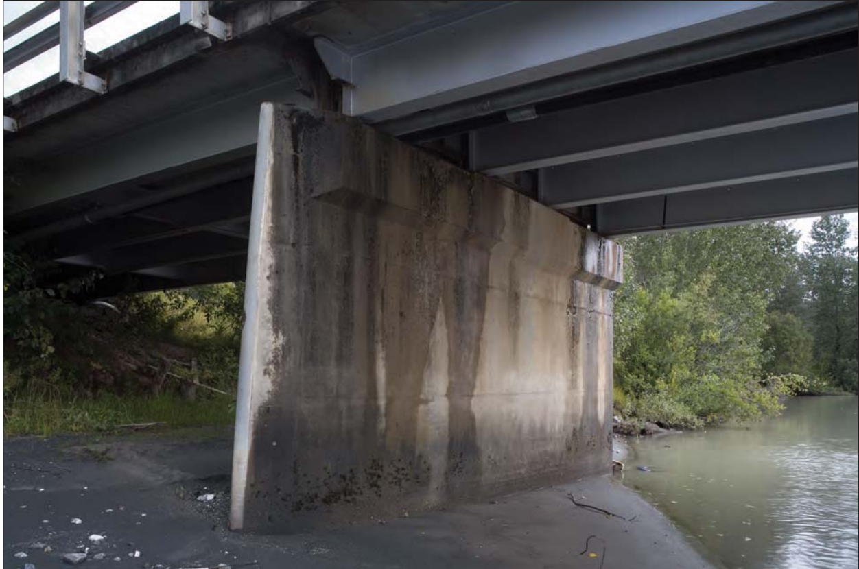
Figure H-14. Upstream end of one of the concrete piers with a steel face showing the short channel sections welded to the stringers to support the curb.
