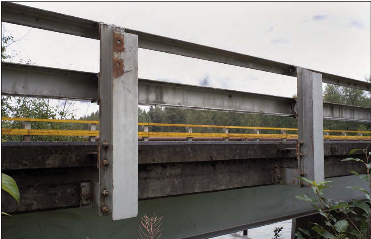
Figure H-17. Safety railings and posts mounted to the concrete curb.
