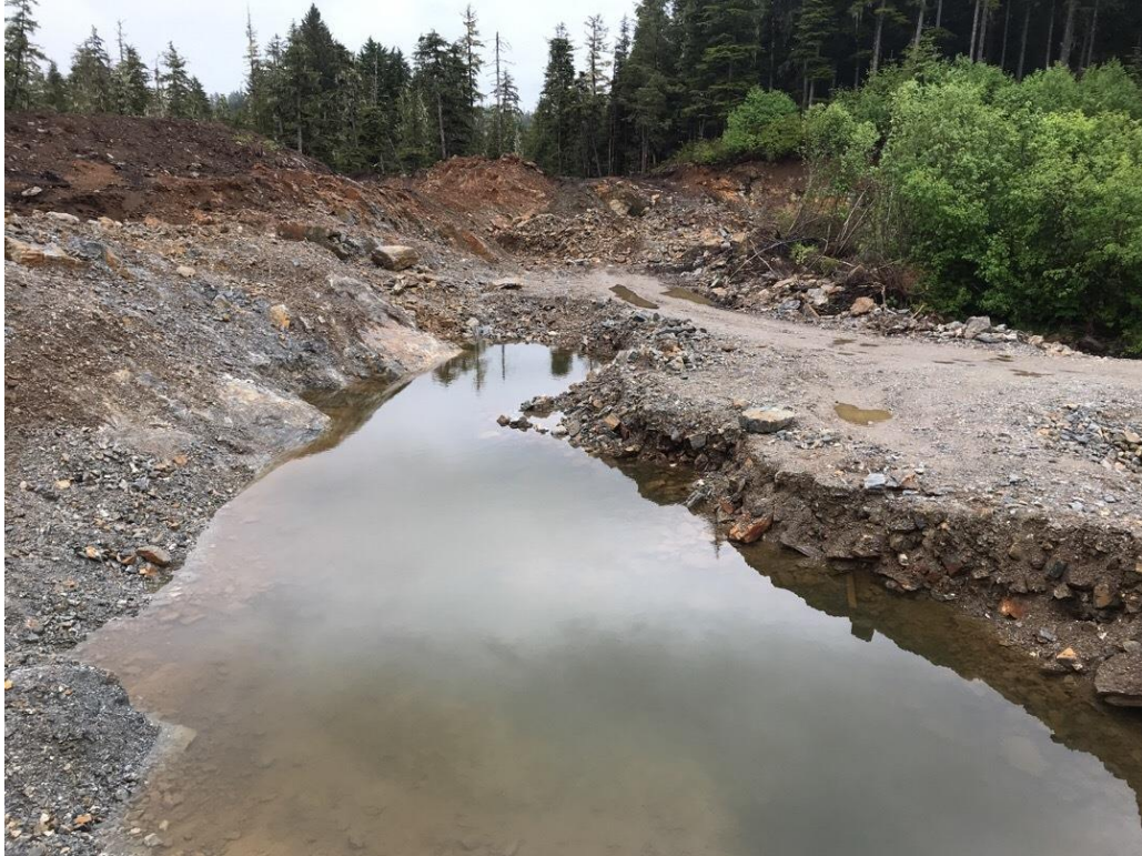
Photo: 31 Ponded surface water within excavated portion of rock quarry (Wetland M) located along Killisnoo Road, looking east (2018)
