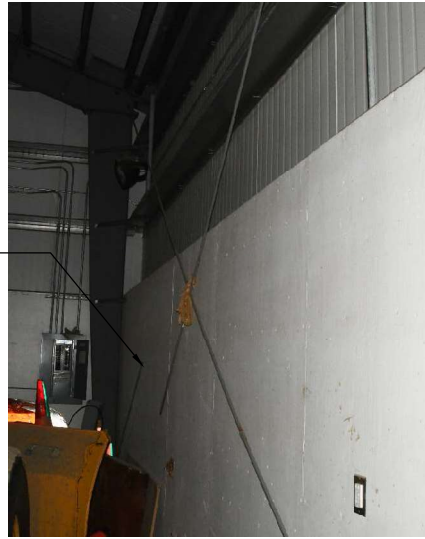
F TENSION ROD COUPLING SREB #1 SCALE: NTS
